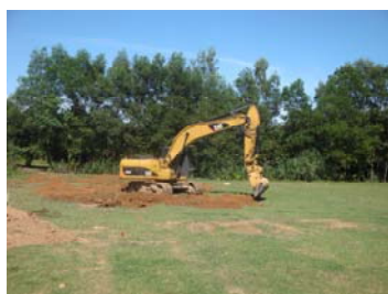
Caterpillar 320 allows for mechanical excavation to reach buried ordnance much faster.
